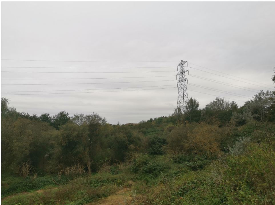
Plate G.1 Looking west to Pylon PAB18, from south-east of the pylon
